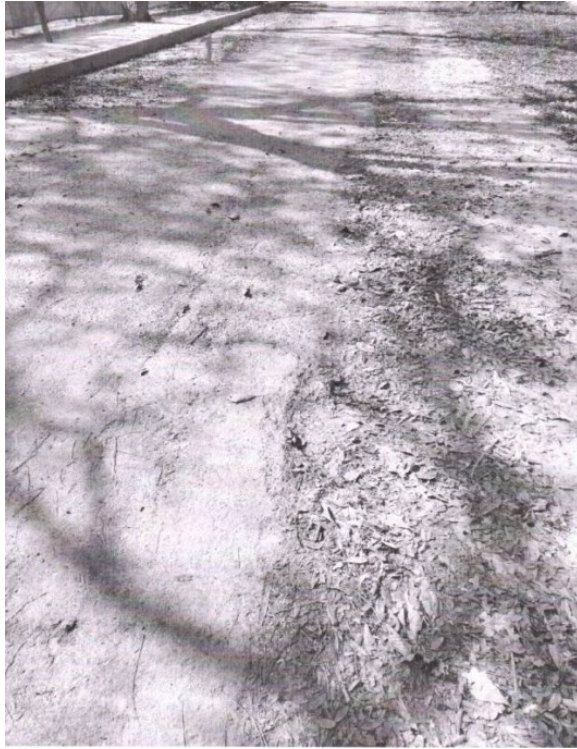
Figure 12: Fig: Rotting on road in main road residence area lane 33
